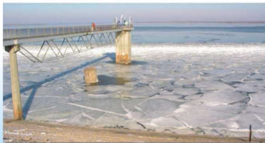
Fly Ash dyke
